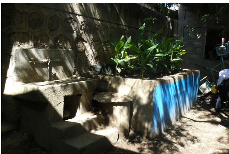
Figure 2-2. Image of the hand WASHing facility and planted reed bed filter
