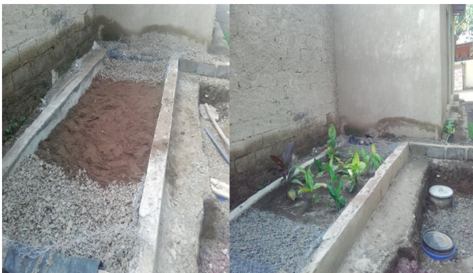
Figure 3-2. Grey water treatment system at the Kidus Kora'an school
