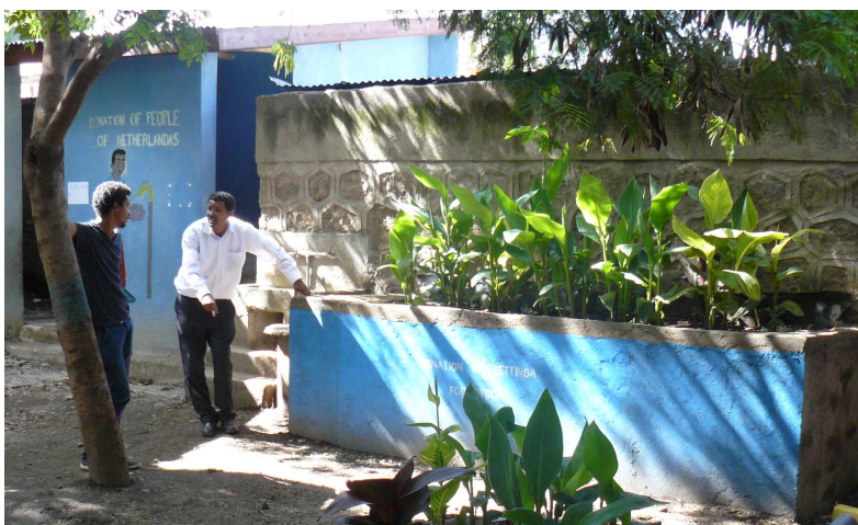
Figure 2-3. Image of the renovated toilet facility (left behind) and the planted reed bed filter
